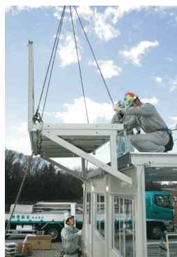
⑤ Walkway is installed from the rooftop of the first-storey
