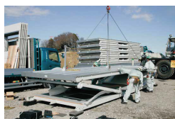
② Lifting the roof
