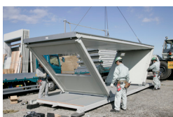
③ Erecting the columns
